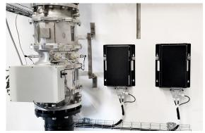
Atlantium's RZ300 systems for IPN protection have been effectively applied in Norway, Scotland, Canada and Chile. The advantage of the wide-germicidal wavelength of the Atlantium medium-pressure lamps enables compact and effective installations for water biosecurity.
